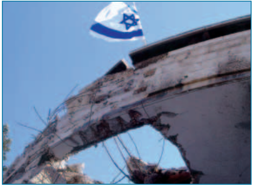
Damaged post office on Rebov Hanevi'im
